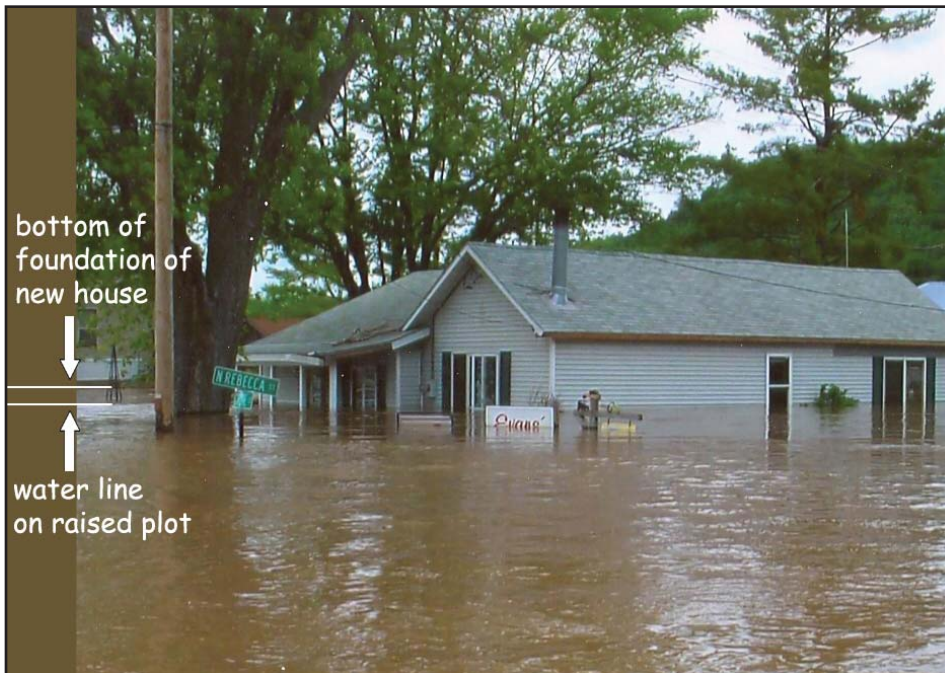
During the 2007 flood the Evans' lived in this house. Their new home is in the background at the left of the photo, protected from damage because of mitigation measures.
