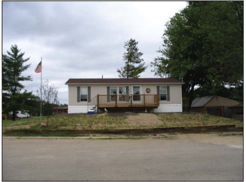
Elevated on approximately six feet of compacted fill, the Evans' home stands dry and undamaged after being tested in the summer 2008 floods.
